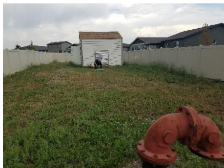
Image 1: Control Building Looking North
