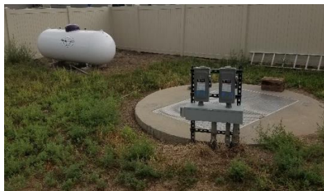
Image 3: Wetwell Exterior & Fuel Tank
