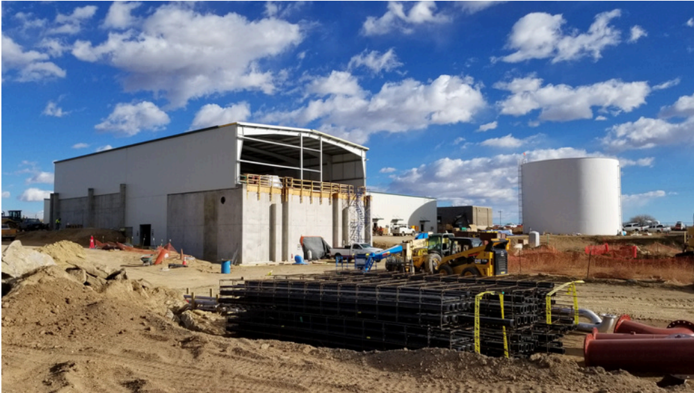
Photo of the Water Treatment Plant under construction.
