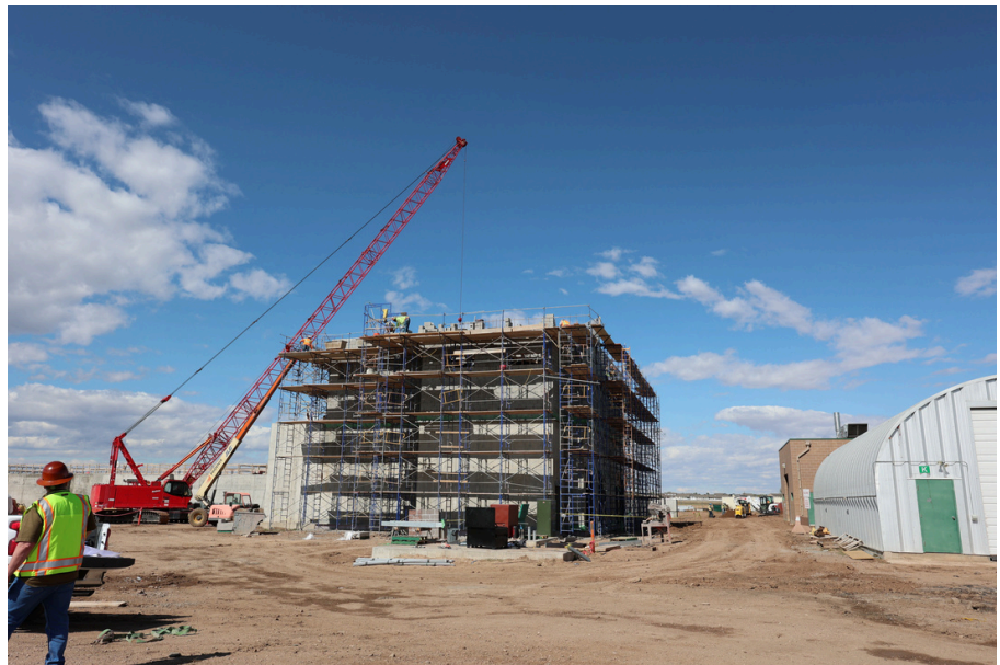
Photo of the Wastewater Treatment Plant under construction.
